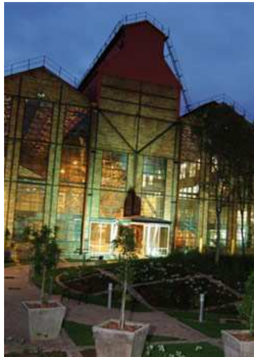
Conserving the building
